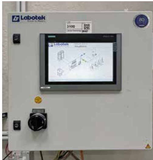
The Labonet control system visualises all the paths taken by the powder from the silo and the granulate from the big bag to each individual extruder.
