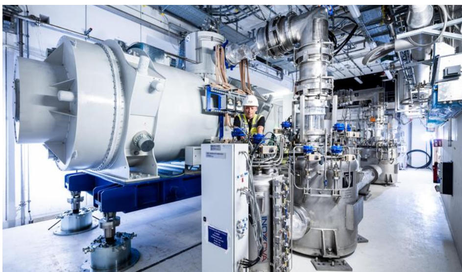
Figure 75: Installation of Super-FRS local cryogenic branch T and sc multiplets.
