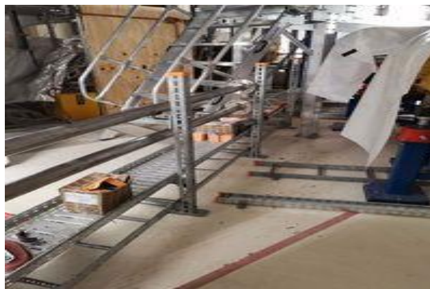
Figure 98: Machine trays and final laying in T1S1 (connection GSI-FAIR).
