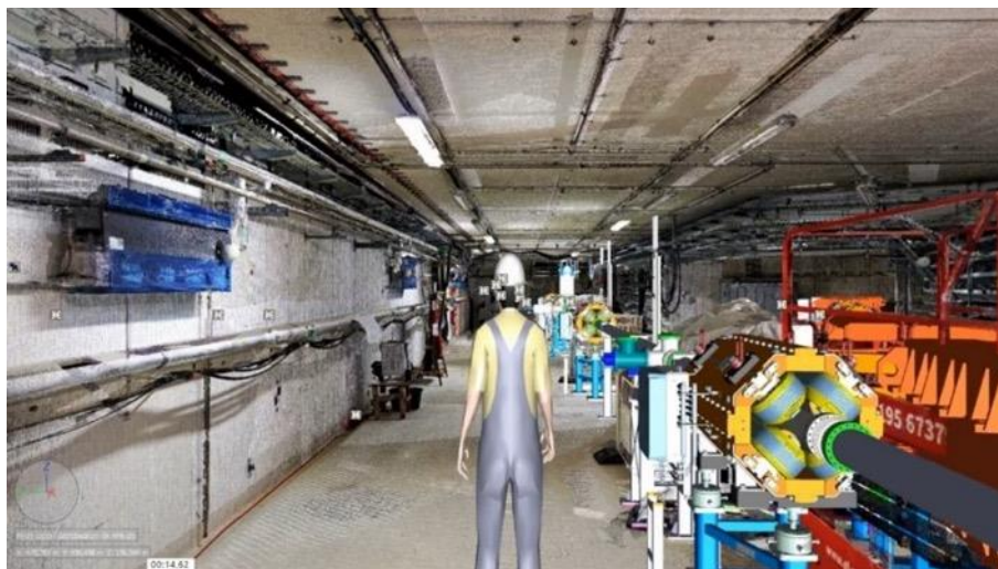
Figure 94: Superposition of CAD model and coloured 3D scanned points in the “High Energy Beam Transfer” (HEBT)
