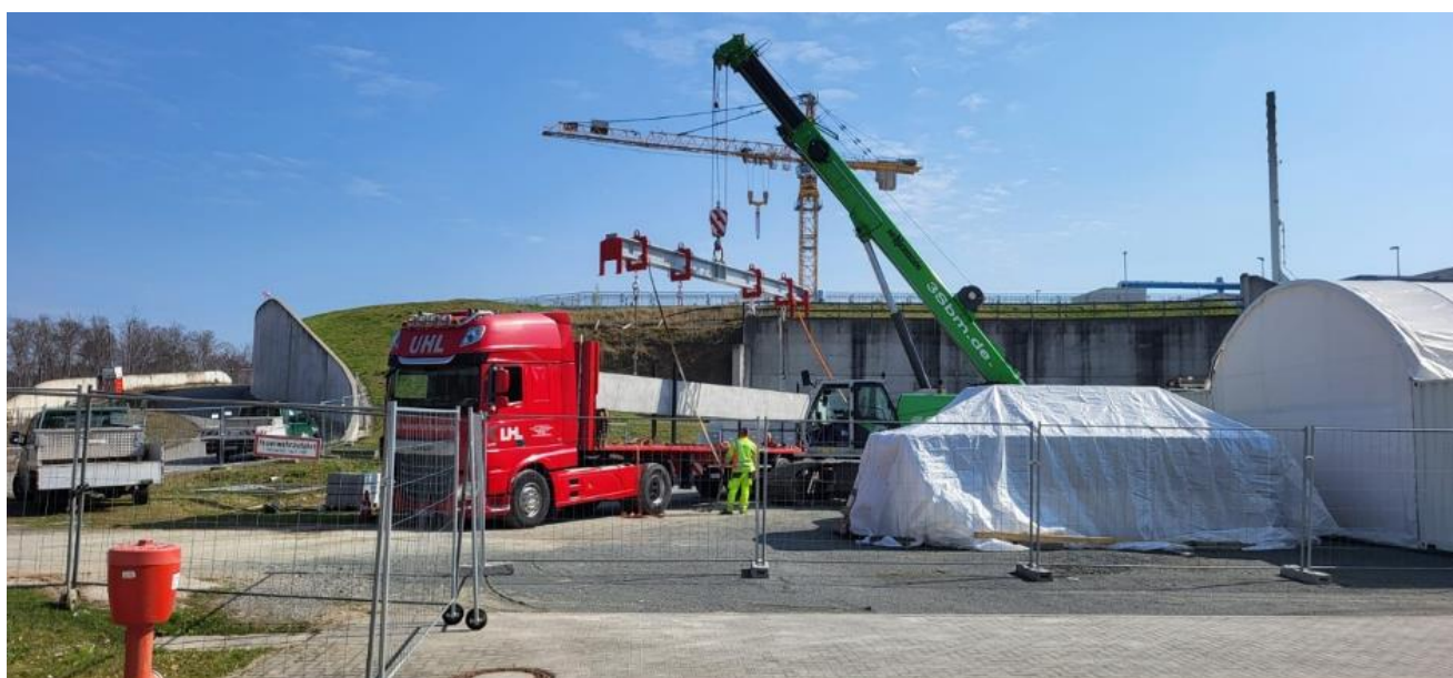
Figure 77: Shielding enhancement of the SIS18 extraction area by means of hematite beams.
