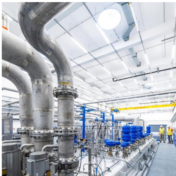
Figure 74: Cryo building under commissioning.
