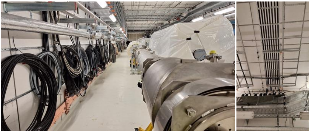
Figure 96: Cable laying in SIS 100
