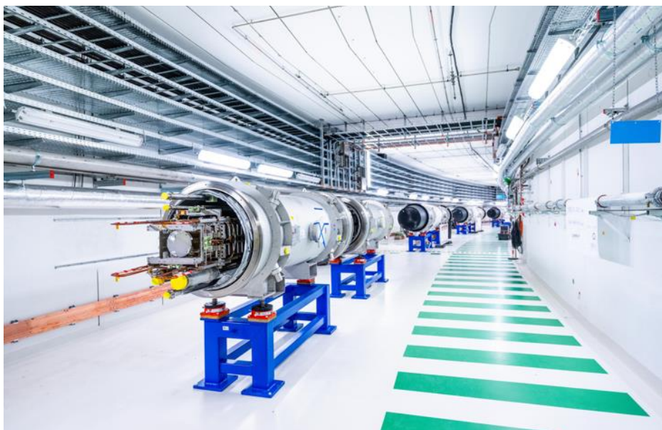
Figure 76: SIS100 dipoles positioned in the tunnel
