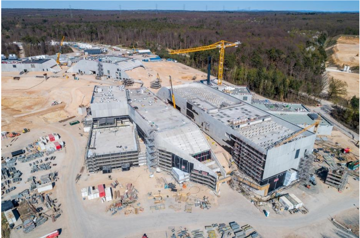
Figure 71: View on FAIR construction Site in April 2025
