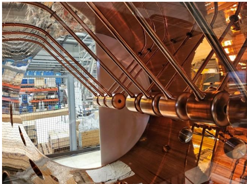
Figure 112: View into cavity section Alla-1 with hanging drift tubes at the GSI Testing Hall (TES).
