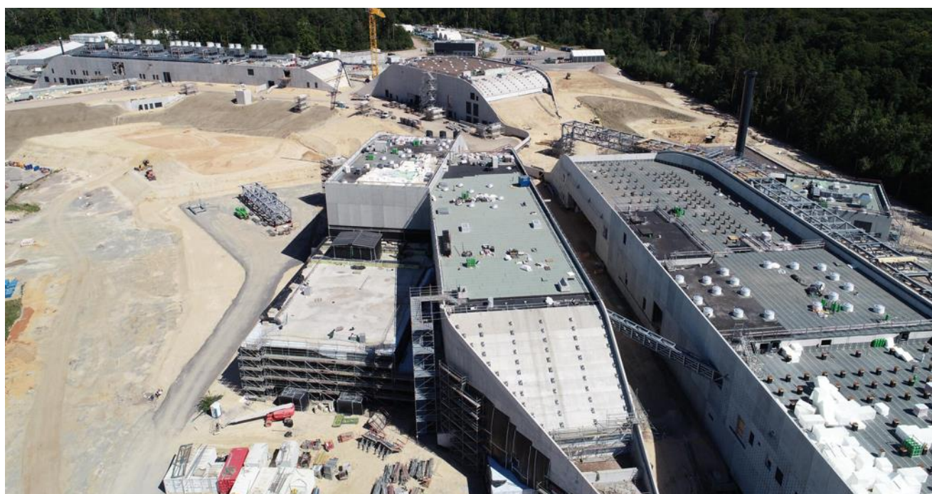
Figure 73: Overview of south area with NUSTAR building on the right, APPA building in the middle, S-FRS & Transfer buildings in the background.
