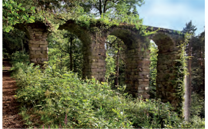
Abbildung 61 — Derbyshire, Chatsworth House, Aquädukt
