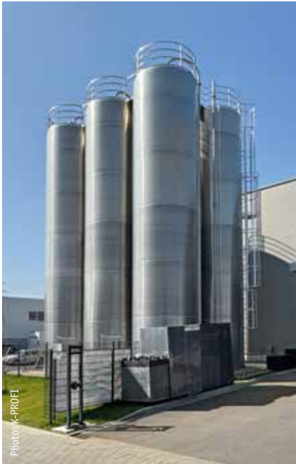
Six brand-new silos from Siloanlagen Achberg, each with a capacity of 78 m 3 , supply the dryers installed by Labotek with polycarbonate via the shortest route.
