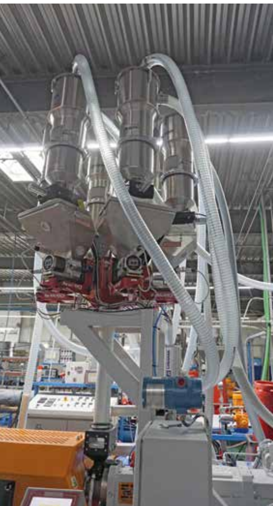
The loss-in-weight 6-fold dosing station feeds the extruder, which runs underfed and produces foamed PE profiles.
