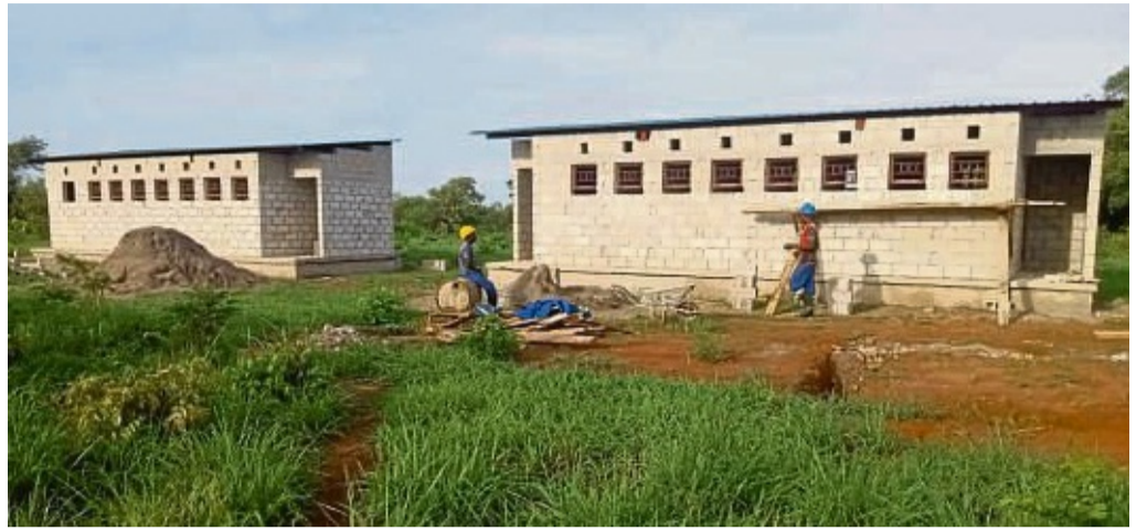
Schulbau in Sambia.
