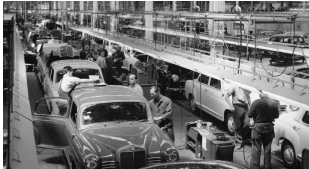
Figure 101: Automotive assembly line: A typical flow shop (Image Unterberg, Rolf under the CC-BY-SA 3.0 Germany license)
