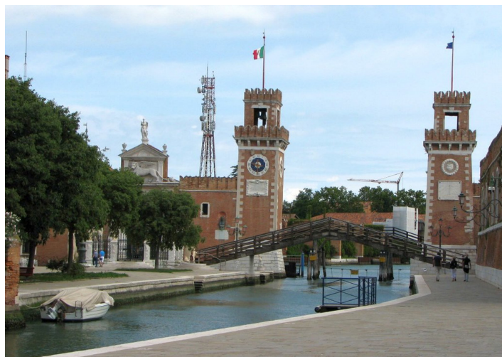
Figure 135: Water gate of the Arsenal of Venice (Image Roser)
