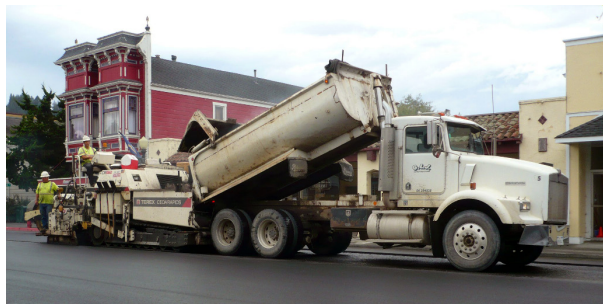
Figure 402: Street Paving (Image Ellin Beltz under the CC-BY-SA 3.0 license)
