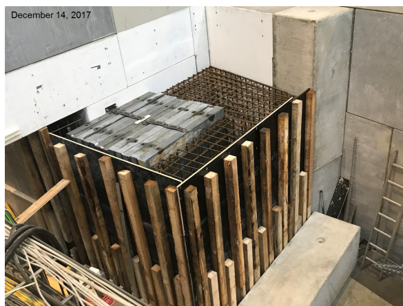
Figure 6: The Iron core of the beam dump is prepared for concrete pouring.
