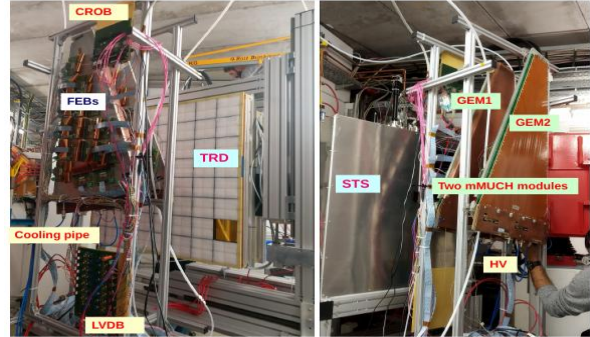
Figure 2: Picture of the detector installed inside mCBM cave. Viewing downstream(left) and upstream(right)
