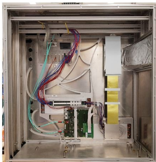
Figure 1: mSTS enclosure with downstream wall removed.
