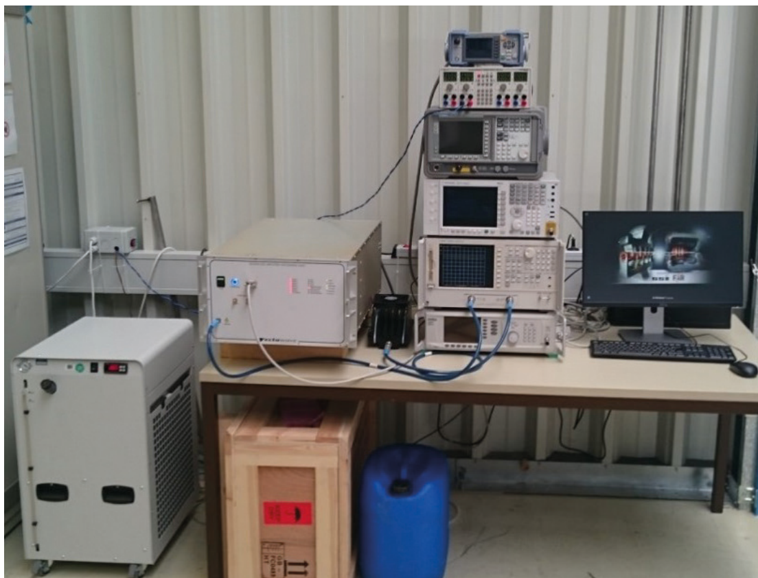
Figure 74. GSI test stand for the SAT of the power amplifiers.
