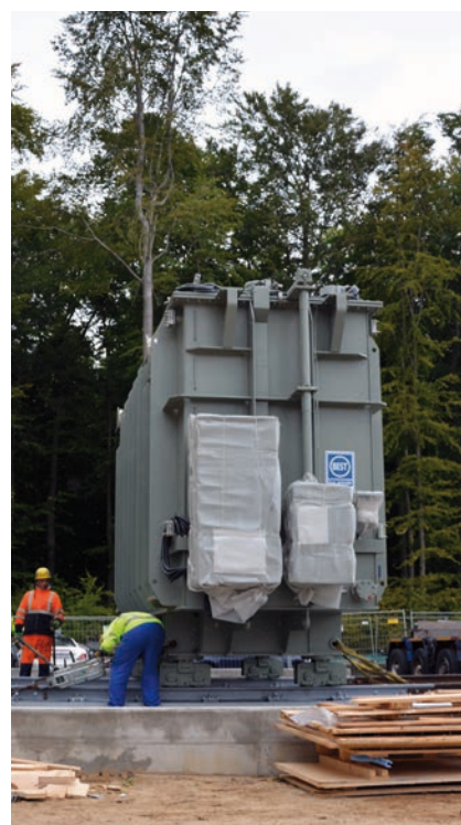
Via rails the transformers are put into position. The transformers are moved with pulleys and muscular strength.
