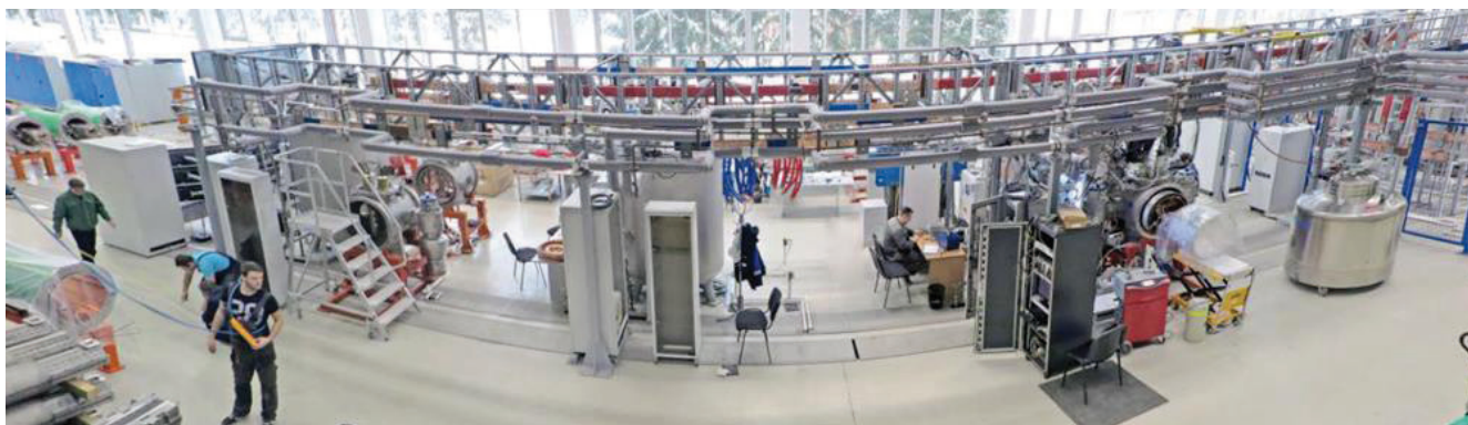
Series testing facility at the Joint Institute for Nuclear Research (JINR) in Dubna, Russia, for superconducting magnets of FAIR and NICA.
