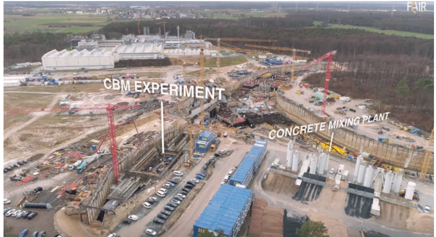
Visit the large construction site of FAIR via drone flight.
