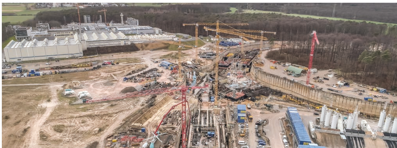
The development is progressing: On the right side the northern part of the construction field with the tunnel for the large ring accelerator SIS100, in the background on the left side the existing GSI buildings, in front of it a part of the southern construction field, which is now being further developed.
