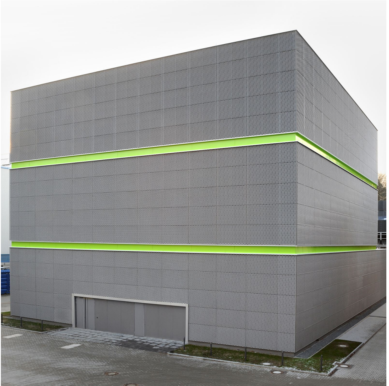
Outside view of the Green IT Cube on the GSI/FAIR campus.
