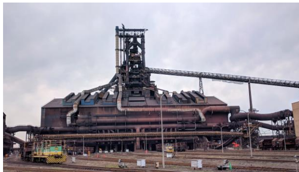
Figure 336: Nippon Steel Yokohama (Image Roser)
