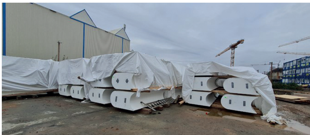
Figure 93. Lateral iron shielding block at the FAIR site ready for installation in Super-FRS target building.
