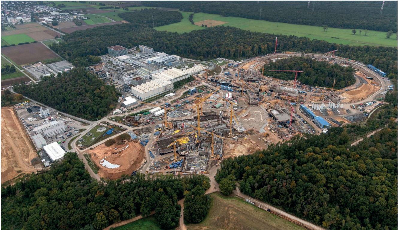
Figure 87. View of the construction field as of October 2021 (GSI, D. Frentz).
