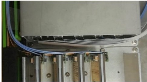
Figure 1: Photo of a mockup illustrating the narrow gap between the FEB boxes available for cabling.
