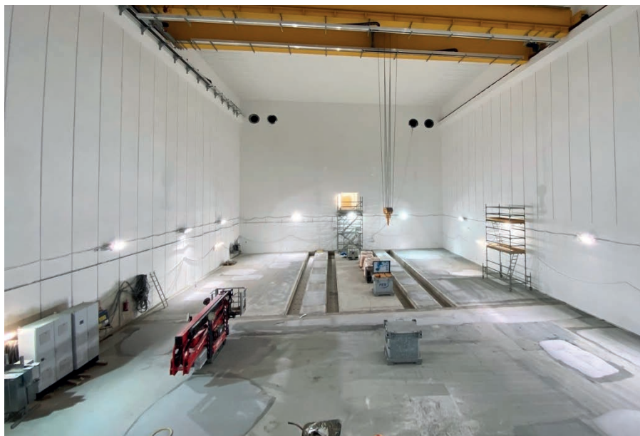
Figure 83. View on FAIR construction Site in CBM Cave December 2022.
