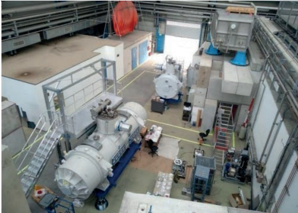
Figure 88. Running pre-assembly of FoS SM and FoS LM at GSI “target hall”.
