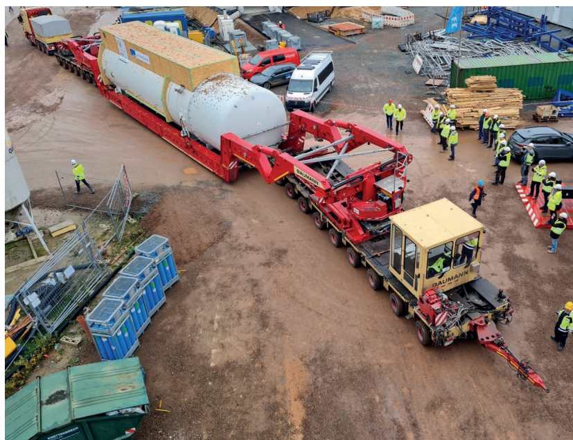
Figure 94. Delivery of the cold box CRYO2 to FAIR.
