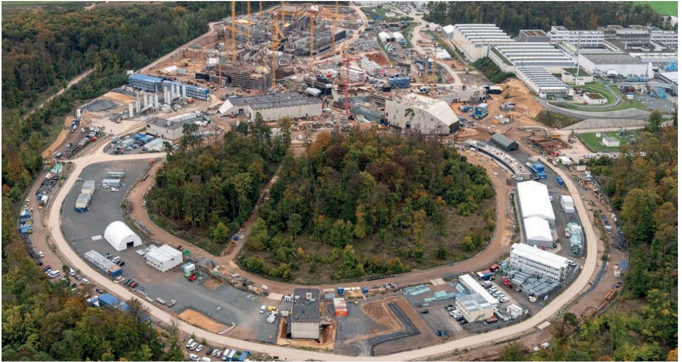
Figure 82. View on FAIR construction Site in CBM Cave December 2022.
