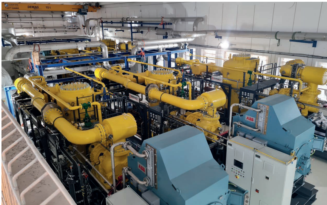
Figure 95. Kompressor system for CRYO2 and CWU.
