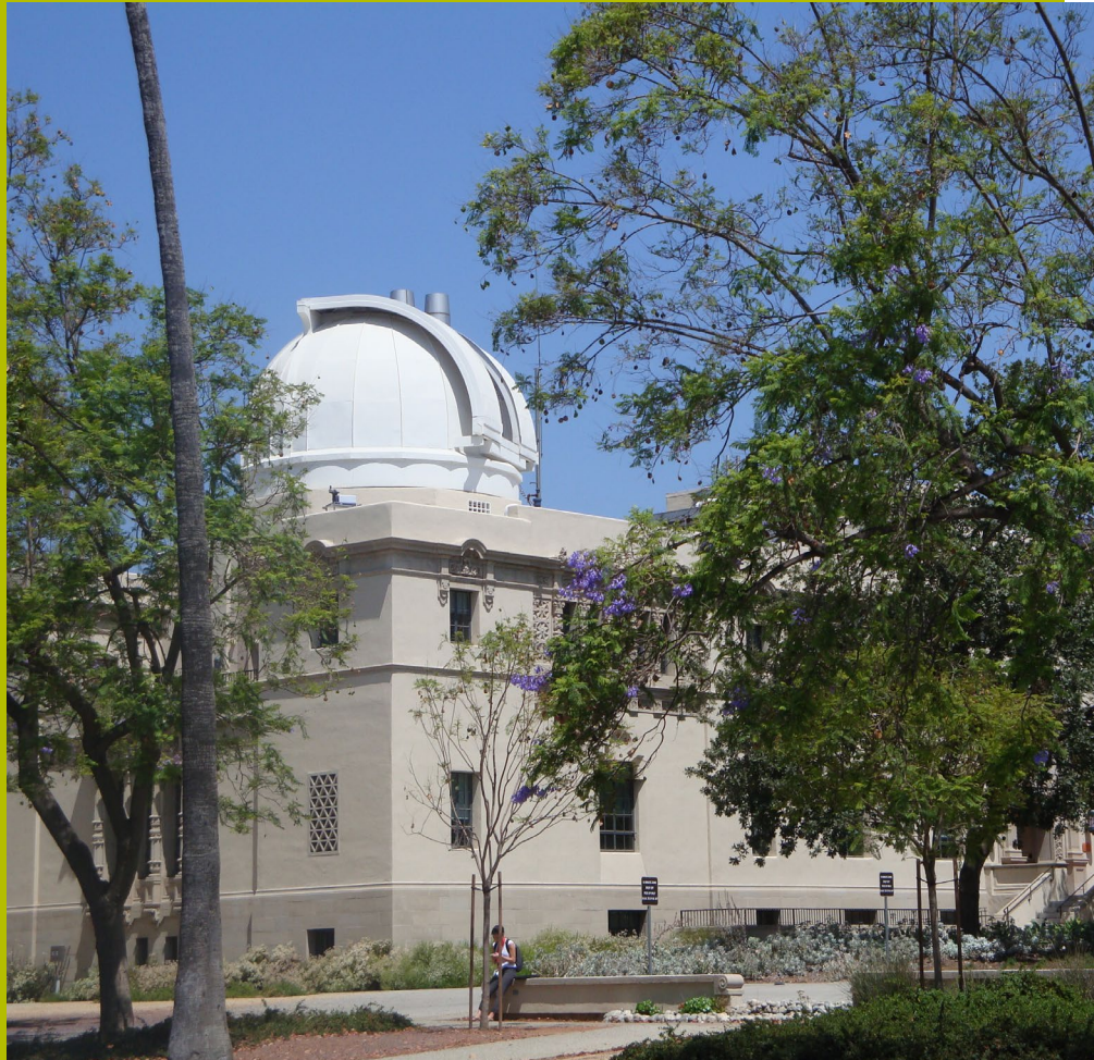
▲ Foto 2.11-1: TCCON-Observatorium am California Institute of Technology (Caltech) in Pasadena in den USA
