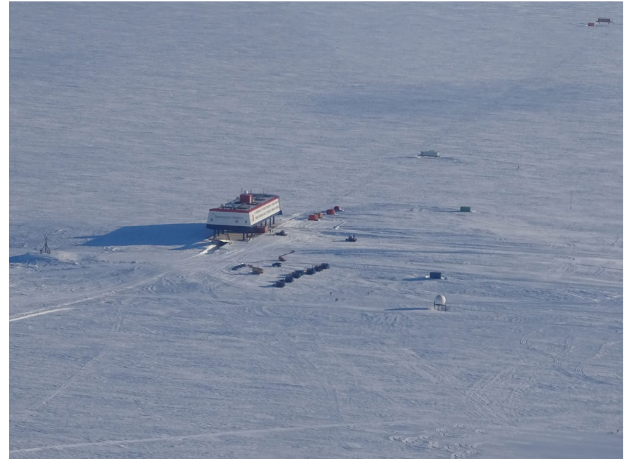
▲ Photo 6.1-1: Neumayer III station (70° 40' S, 8° 16' W) on the Ekström Ice Shelf in December 2018. The measuring instruments of the observatory are situated 350 m to the south-west of the main building. Some others are installed on the roof of the station. The station's trace gas measuring site is situated 1,500 m further south; it can be seen in the top right corner of the picture.
