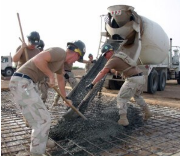
Figure 225: Pouring concrete (Image Edward Miller in public domain)
