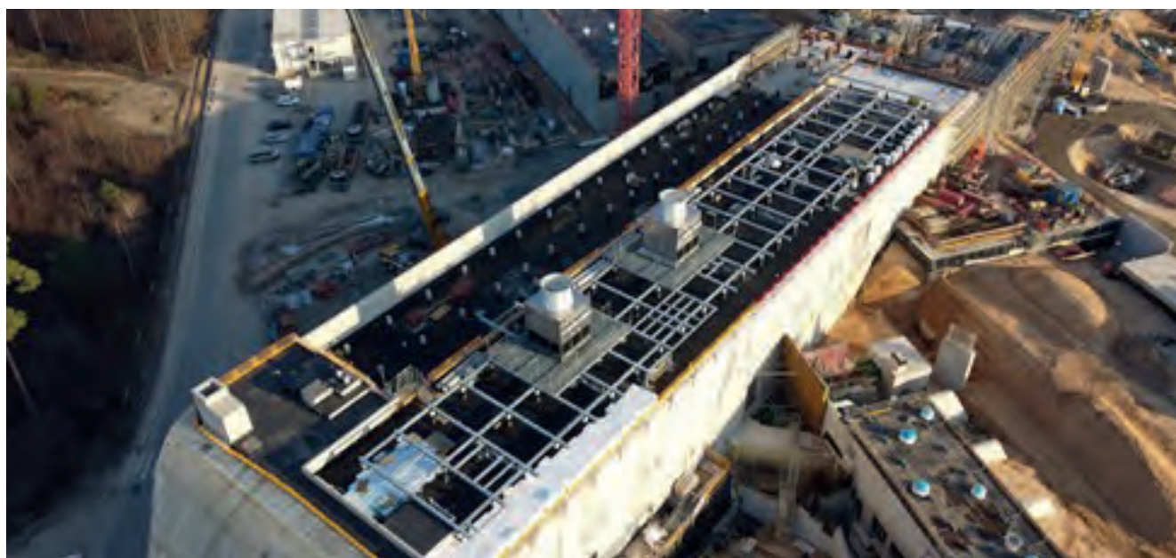
Figure 113. First 2 air coolers were installed on the building H0719A
