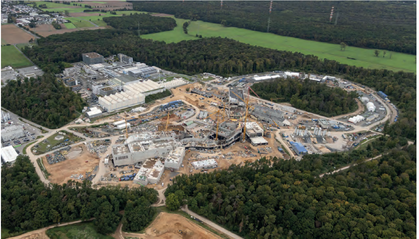
Figure 111. View on FAIR construction Site in October 2023
