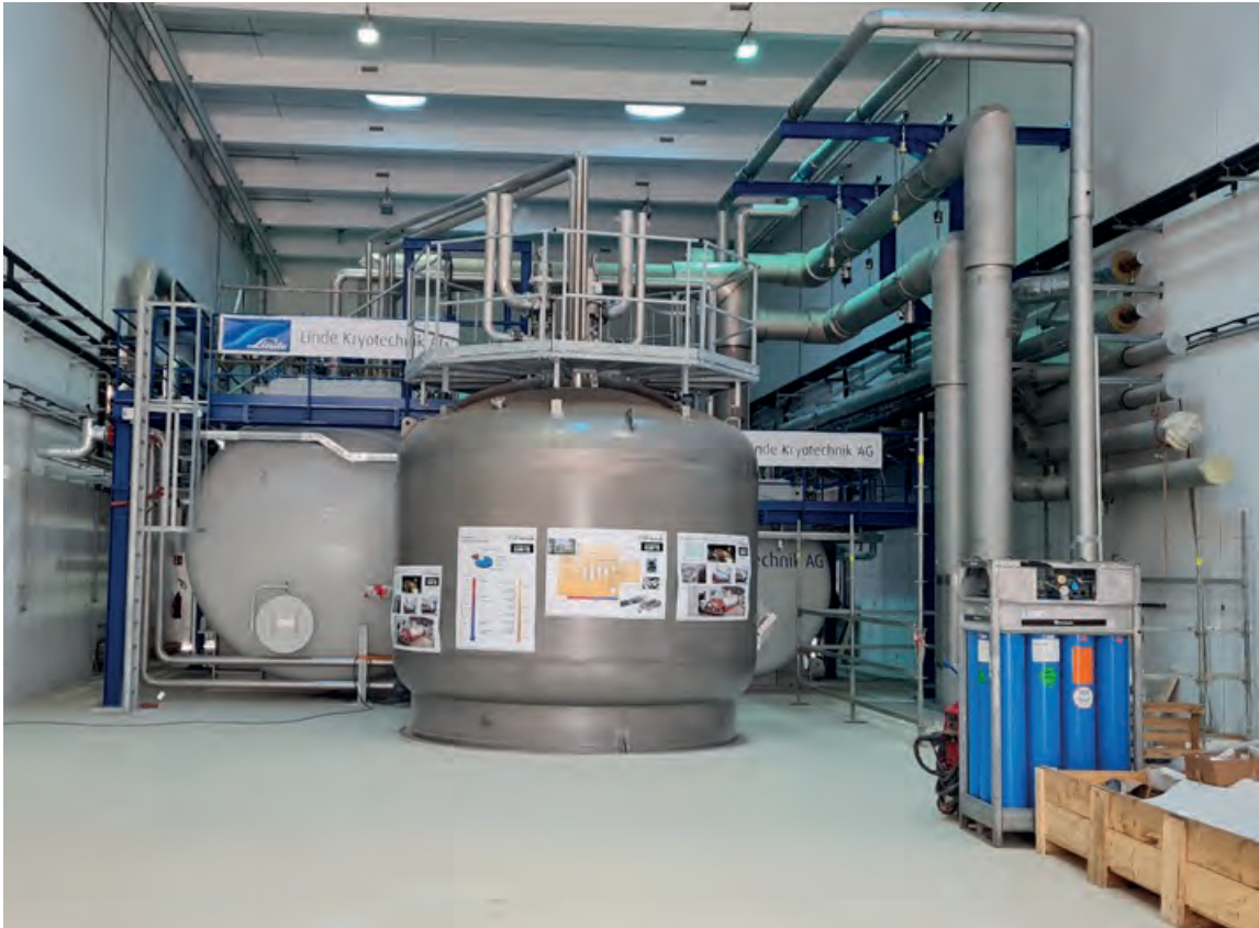
Figure 123. Cold box and DB3 installation after mechanical completion
