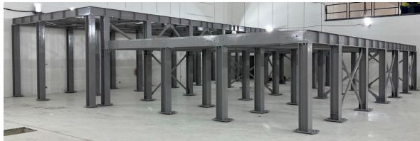
Figure 2: Finalized UP steel construction installation in CBM cave.
