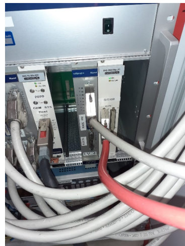
Figure 9: Low Voltage and High Voltage supplies located at the cave entrance.
