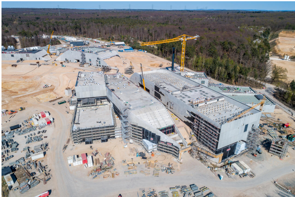
Figure 58: View on FAIR construction Site in April 2025
