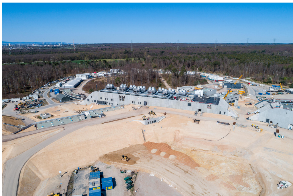
Figure 60: Air coolers installed on the main transfer building H0719A
