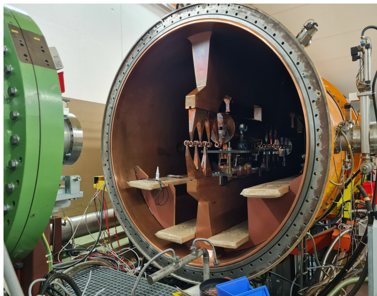
Figure 96: View into IH1 with construction installation
