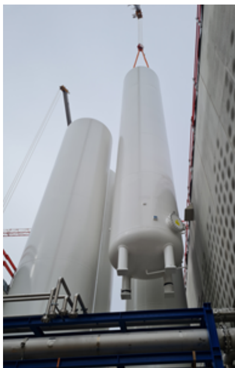
Figure 80: Erection of the first 6 helium tanks
