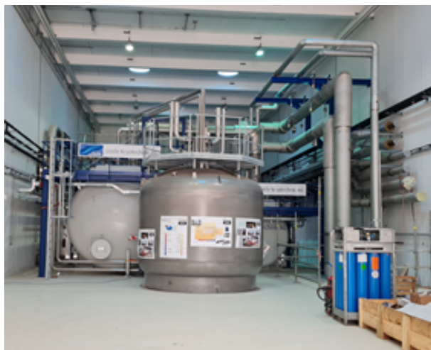
Figure 78: Cold box and DB3 installation after mechanical completion
