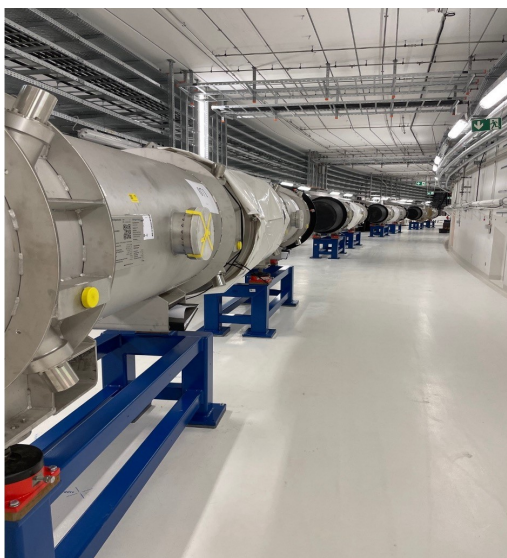
Figure 63: SIS100 dipoles positioned in the tunnel
